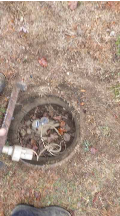
16: The domestic water supply main shut-off valve is located at manhole by the road.
