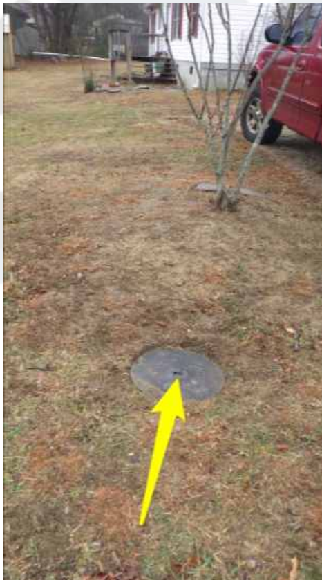
16: The domestic water supply main shut-off valve is located at manhole by the road.
