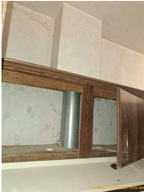
41: Ventilation: Exhaust ducted to the exterior
